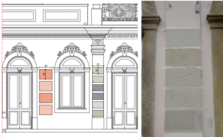
Figure 4: Wall Paintings testing
