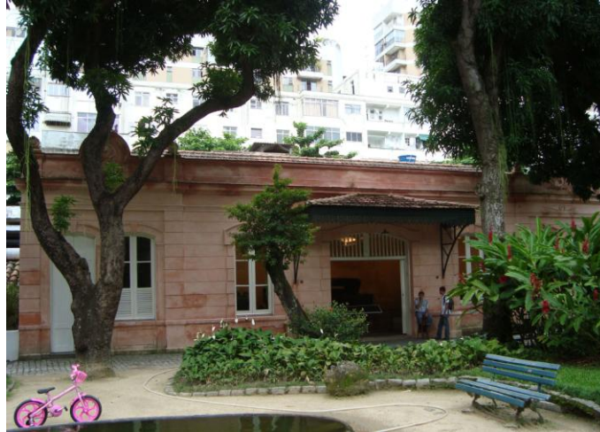
Fig. 4 Stable façade restored with lime plaster two years after the intervention.
